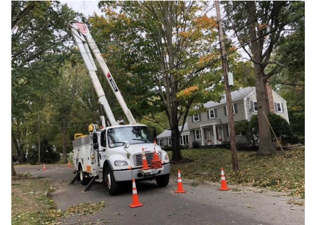
Fig. 1. Distribution system repair.
